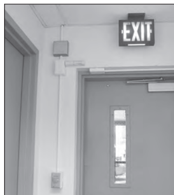
Typical applications for 700 Series Raceway.
